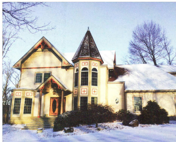
Snowmelt patterns provide exterior signs of energy loss.
